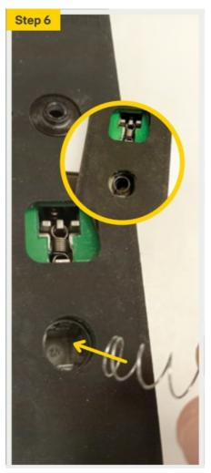
7. Feed the External body cable through the lock cylinder hole. Place the External body onto the stile, insert the spindle through the lock case, and spindle hole in the External body. A clamp can be used to hold the external body onto the door, in preparation for the next step. Important: Ensure the cable is not pinched and External body is aligned correctly with door mounting holes.
