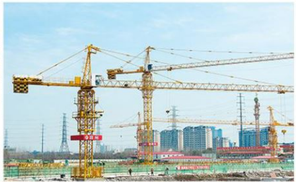
Tower crane site
