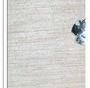
+ Drill six 7mm holes for the Tee Nuts.
