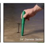
Attach the vacuum attachment to the straight extension of a shop vacuum cleaner hose\* and thoroughly vacuum up the dust in and around the hole.
