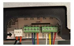
5. Plug the VTech Wiring Harness into the Controller module. Press the connector firmly to ensure it snaps into place securely. Then, restore power to the PTAC/PTHP.
