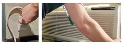
2. Using a Philips screwdriver, remove the cover panel to access the Wired Thermostat Terminal panel.
