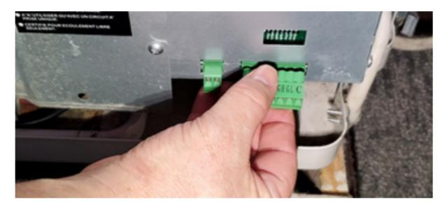
3. Using a precision screwdriver, change the #2 Dip Switch to the UP (On) position. This will enable Wall Thermostat control.
