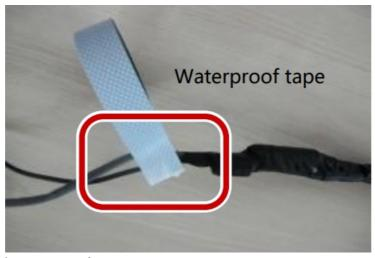
6. Protect the tail cables using waterproof tapes.
