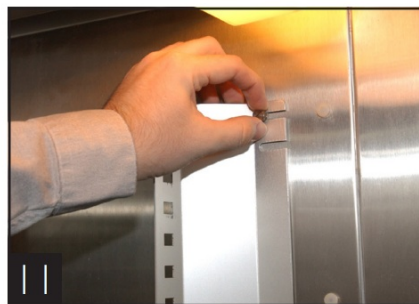
11 Pilaster installation two and three door models (middle of wall in rear of cabinet)
