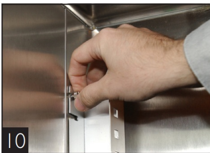
10 Pilaster installation (side wall of cabinet)
