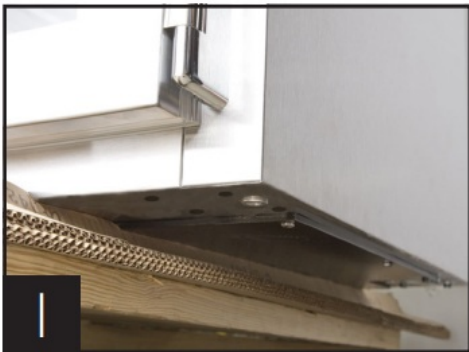
Slide packing material under the unit.
