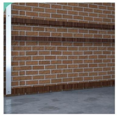
3. Install starter bar, ensuring that it is at least 30mm from the ground.
