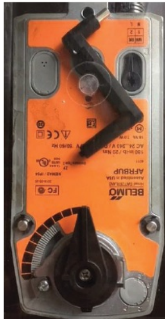
Figure 6. Powered open position (cooling cycle)
