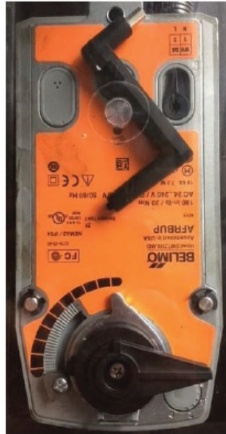
Figure 5. Spring closed position (bypass cycle)
