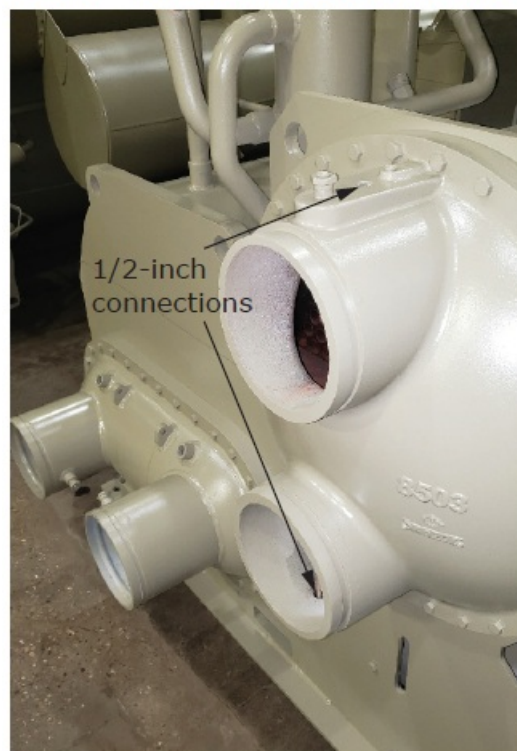
Figure 3. Cast - \frac{1}{2} inch NPTI port (threads directly into port)
