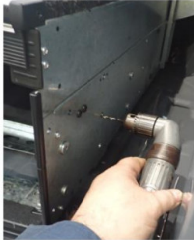
Pilot drilling of marked hole locations
