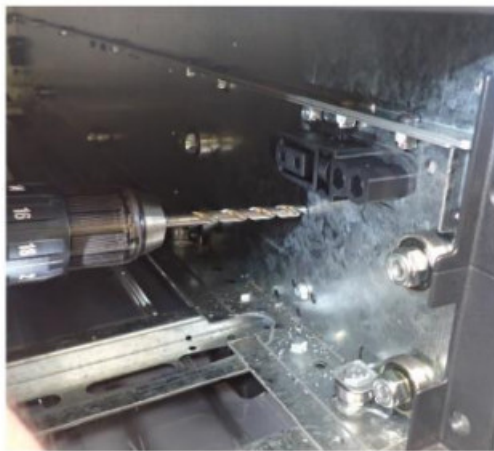
Drill pilot drilled holes to specified diameters
