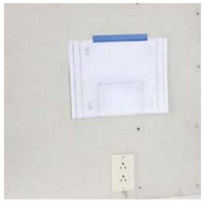
2. Install drywall anchors (4) and screws (4). Tighten screws within 1/16" of anchor.
