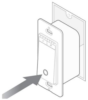
6. Attach the wallplate and turn on the circuit breaker. Then the wiring is finished.
