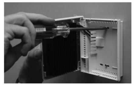
6. Reinstall the front part of the thermostat on the mounting base and tighten the screw at the bottom of the unit.
