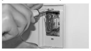
5. Take the wires from the wall through the hole at the base of the thermostat and connect them using the supplied solderless connectors. When making the connection with aluminum wire, make sure that you are using connectors identified CO/ALR. Please note that the thermostat wires do not have polarity. Therefore, the way they are connected is not important.
