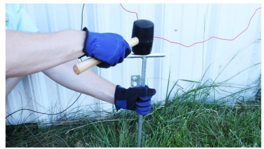
• Try to get the ground rod into the ground as far as you can without obstructing the area where the clips will go
