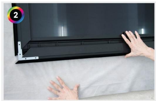
3. Insert the vertical frames into the outer horizontal frames at the same time.
