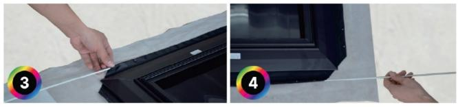
4. Adjust the inner frame to align the stickers of the screen. Place the screen in the middle of the inner frame and hook the screens to the frame. This is much easier to accomplish with a second person helping (as pictured). Start from the middle springs and connect the corner springs using the pull hook.
