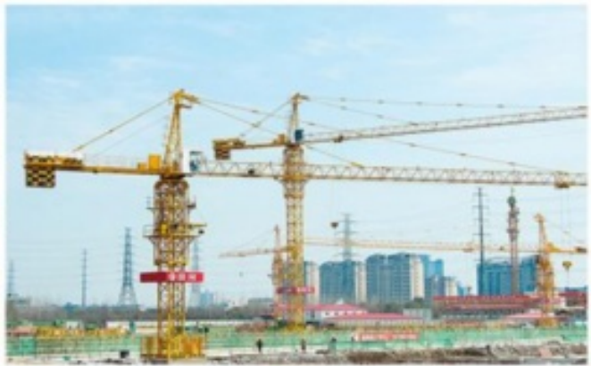
Tower crane site
