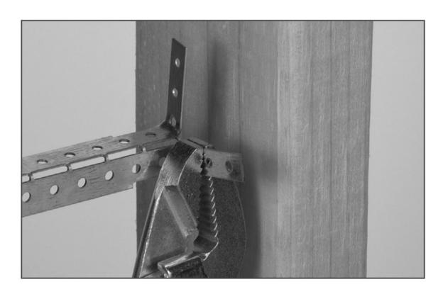
Bend in both tabs to fit the bracket inside the stud bay.  $\bf Narrow\ Stud\ Bays$
