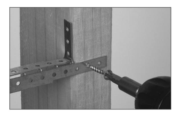
Use screws or nails to secure bracket to either the front or inside of stud. **Inside Stud**
