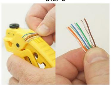
Straighten each wire conductor.
