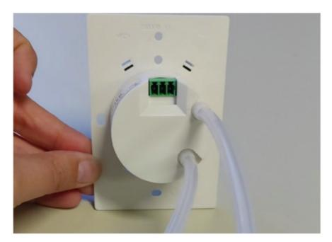
2. Add connector to the in-wall wiring for power and analog output (if required) per section 7.0. Attach the power connector to the Filter Alert and the intermediate tubing to the in-wall tubing.
