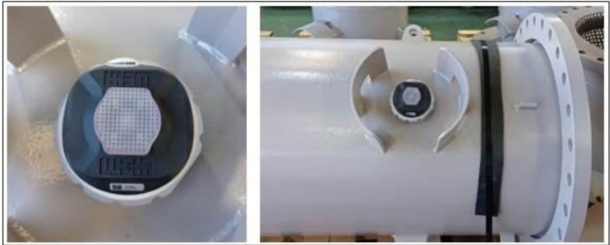
Figure 9. Spool installation
