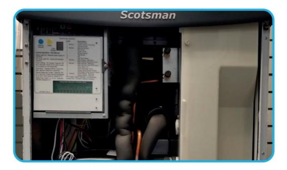
1. Before working on the ice machine, the ice in the bin must be removed. Turn the ice machine power to off or unplug the unit.
