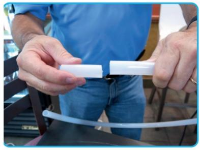
19. Assemble the supply and return fittings to the 90 degree hose barbs using the 2.5 inch pieces of tubing. Installer's Tip: Heating the tubing in hot water eases the installation of the tubing onto the fittings.
