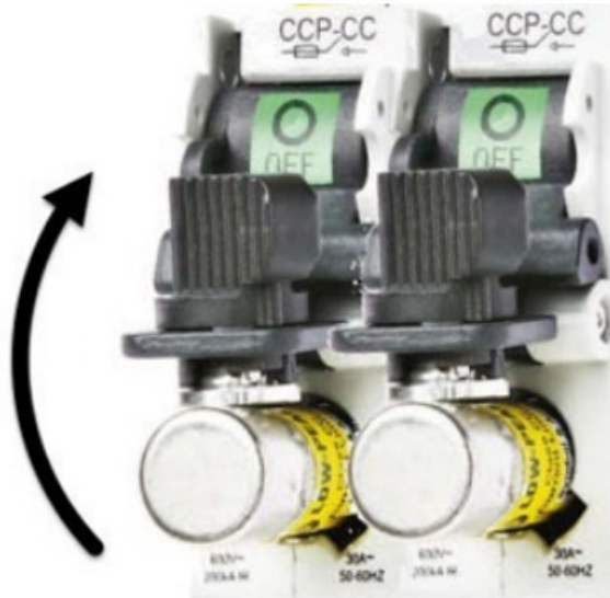
Figure 6 : Opening Fused Disconnect to Replace Fuses
