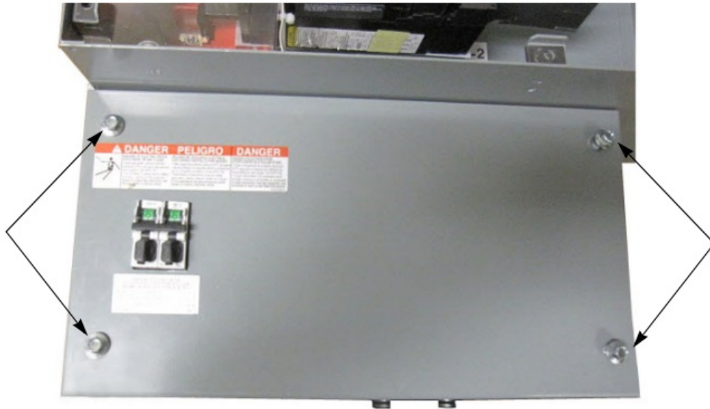
Figure 5 : Removing Cover of Communications Box
