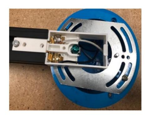
**Step 4.**Place the cover plate over the electrical box and the machine screw and secure it with the white cap; Now installed the live end feed cover plate Figure 2.
