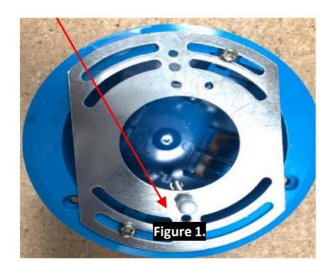
**Step3.**Connect the Live end connector to the track and make all your electrical connections, ensure the grounding conductor matches per image #1.
