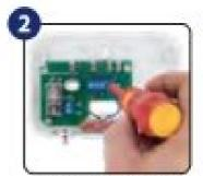
Mount the back housing of the receiver, and then connect wires according to the appropriate schematic for your heating device.
