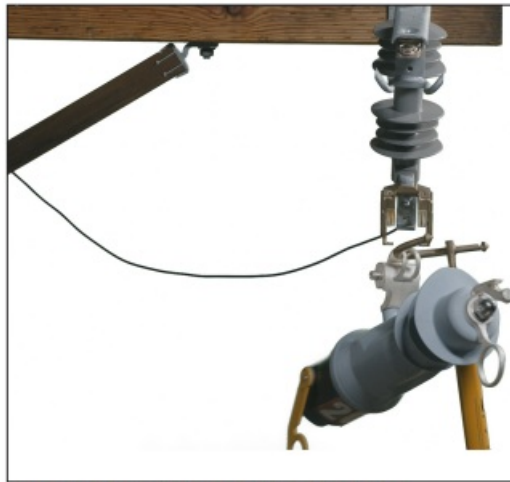
Figure 9. Using a Talon tool during installation.
