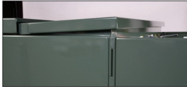
Figure 4. Roof section disengaged from pad-mounted gear enclosure.
