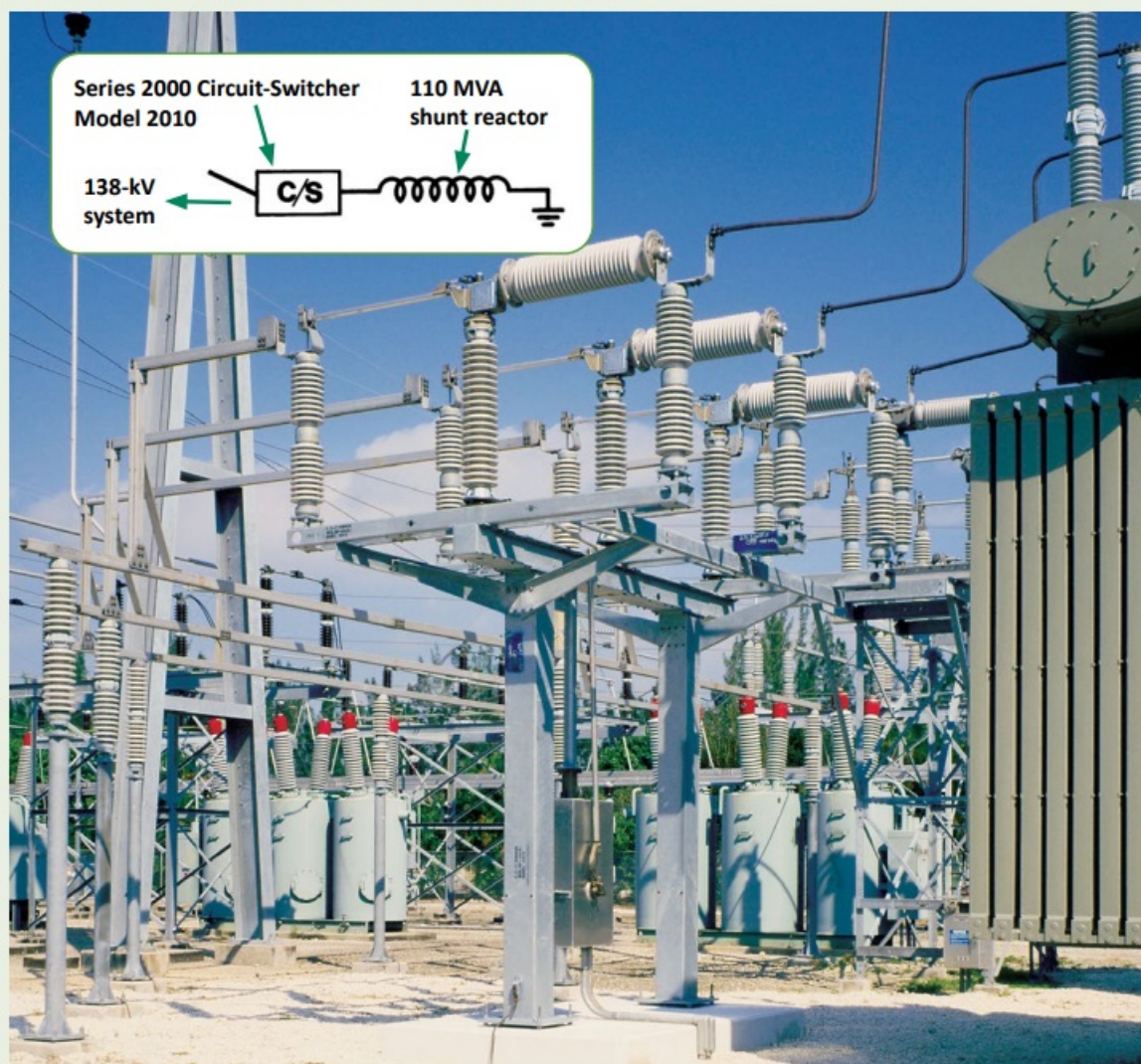
FIGURE 2. A 138-kV Model 2010 Series 2000 Circuit-Switcher with horizontal interrupters and a vertical-break power-operated disconnect, applied for switching and protection of an oil-insulated shunt reactor at a substation belonging to a large southeastern utility.
