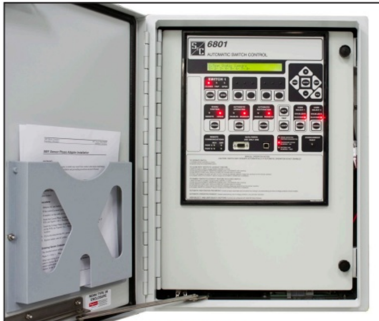
Figure 1. A new 6801 front panel installed on a 5801 control.
