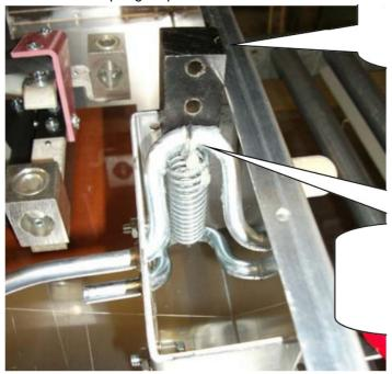
Switches are shipped from the factory with shrink tube or sleeving installed over the turnbuckle. Now is the time to make sure that is in place.
