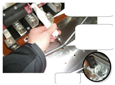
The turnbuckle should measure approximately 7-7/8" when properly adjusted. This measurement is taken from the center of the eyes of the turnbuckle. A visual check of the measurement may should be sufficient as it may be difficult to get an exact measurement when assembled.
