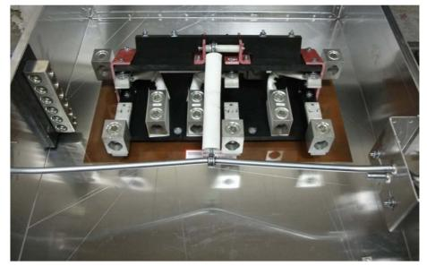
Fine tuning can be done by measuring the distance from the turnbuckle eye on the crank to the back of the switch enclosure. Ideally, this will be equal. The goal is to get equal pressure on the contacts. Small adjustments should be made to meet that goal.
