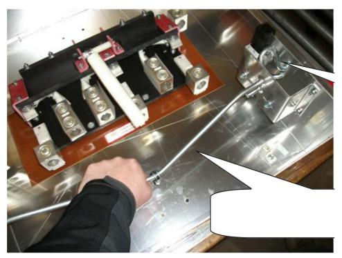
Insert a 1" square block of wood into the space between the crank loop and inside handle bracket to hold tension on the spring.
