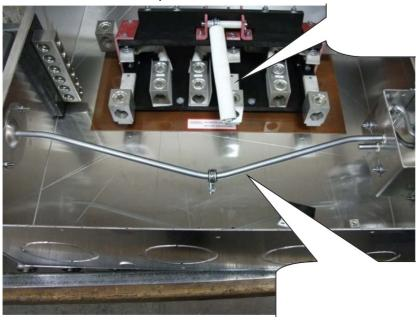
Put the handle crank into the lower position
