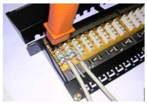
5. Fasten the screws through metal case to hold tightly down for two cable jackets in the same time.
