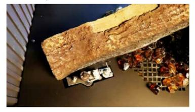
Snip off any strands of wire wool sticking out around the flame rod. These are the most common source of installation problems. These strands can short the flame rod out and cause flame failure errors or pre-ignition flame rod failures.
