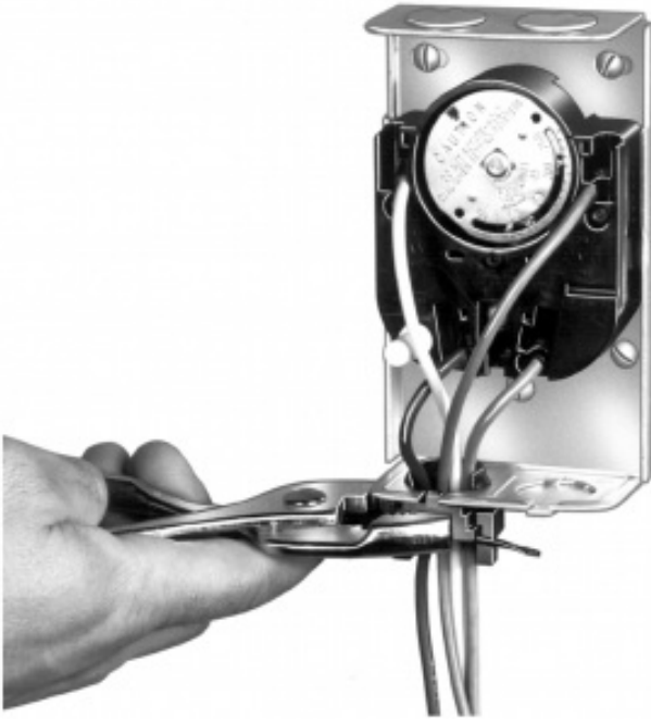
Fig. 8. CLOSING THE STRAIN RELIEF BUSHING.
