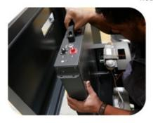
Slide out one battery at a time. Be careful handling as each battery weighs 42 kilograms.
