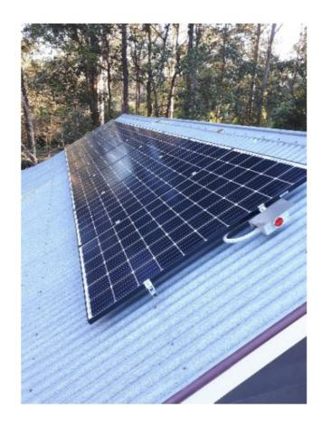
Note that the BlackMax has two MPPTs, so PV panels can be installed facing in two different directions.
