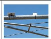
Use the supplied zip ties to secure the Solar Panel assembly and Data Gat eway
