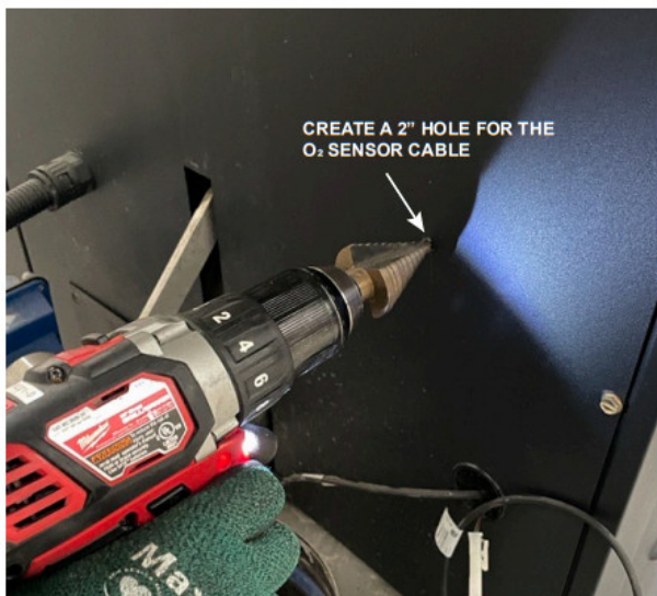
Figure 15. Create Hole for O 2 Sensor Cable
