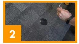
3. Drive the bolt until it compresses the Microflashing®
