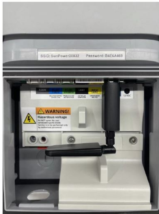
Photo 2.1: The communication module in the measurement meter
