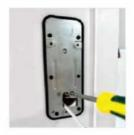
Align the holes of the built-in board and fix them with flat head screws
