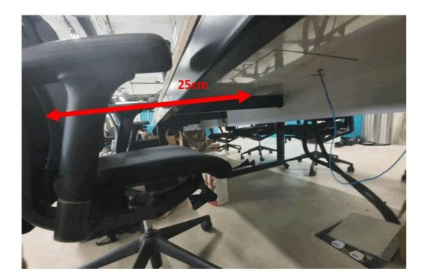
Every BLE Sensor need to be place at every seat correctly. According to the label of the sensor. The Recommended distance of the sensor pointing toward the seats is 25cm.
