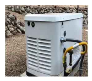
Using a propane backup furnace and tankless water heater allowed Owens to specify an affordable standby generator, since it didn't have to be sized to operate the home's mini-split heat pumps.
