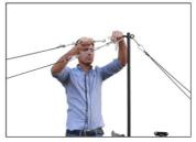
Attach 24ft cable to hook attached on 1st section of the jib and another end with 3rd hook attached to cable guide as shown below.
