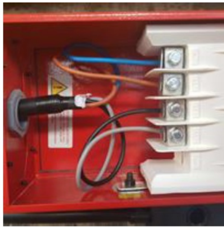
Figure 5. Wiring of Busbar Feeder Unit
