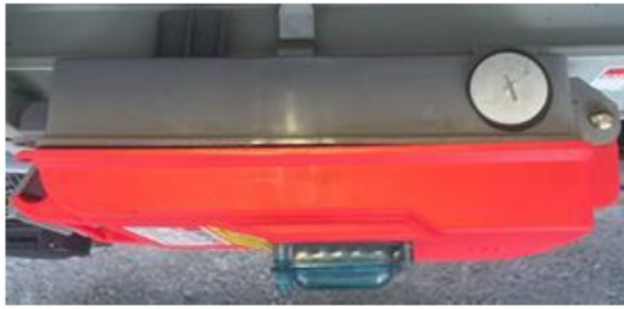
Figure 26. Tap-off Box fitted to Busbar (Top)
