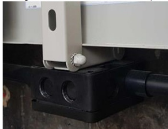
Figure 20. Example Conduit fitted to Data Box
