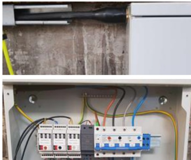
Figure 4. Supply to Distribution Board
