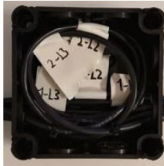
Figure 22. Looped, zip-tied and marked second set of Data cables
