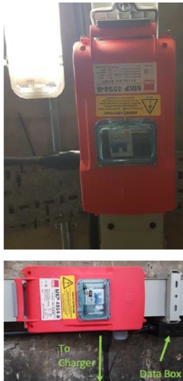
Figure 38. Examples of a Tap-off Box and Data Box fitted to Busbar and feeding a Chargepoint
