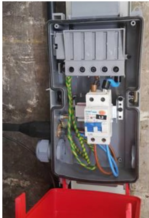
Figure 29. Tap-off Box with L2 connected to RCBO
