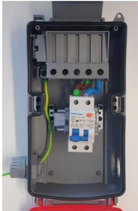
Figure 24. Tap-off Box with L1 connected to RCBO
