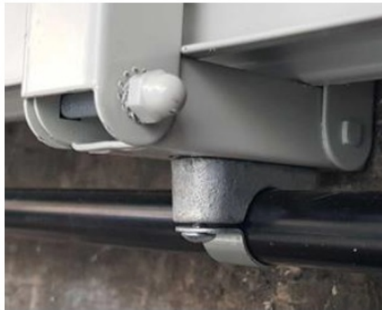
Figure 19. Conduit fixed to saddle clamp
