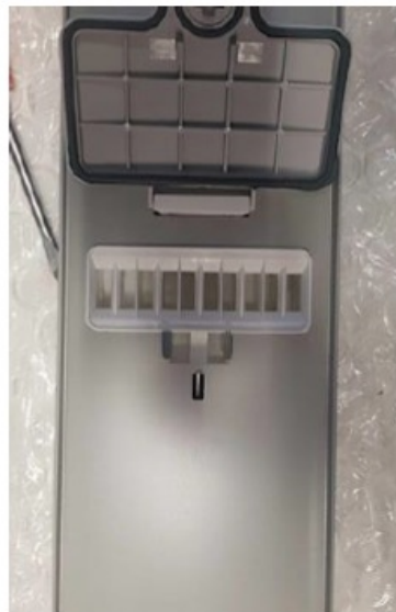
Figure 25. Exposed Tap-off Point, cover to be removed
