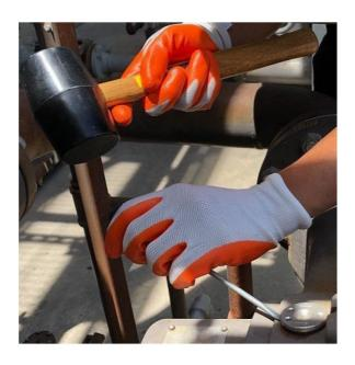
**Step 3:** Clean the Mount by chipping away any leftover epoxy residue with the Chisel/Rubber Hammer. A Handheld Grinder can also be used to clean the Mount.
