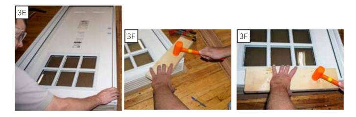
F. Starting on one head and jamb corner; use a block of wood and mallet to tap the frame clad onto the molded nose. Make sure the clad is fully seated onto the molded nose with no gap between the clad and composite frame material.
