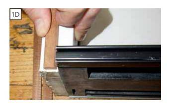
E. Use the provided template to position the molded nose correctly with the arrows pointed toward the door panel. Near one end, insert a staple next to the template.
