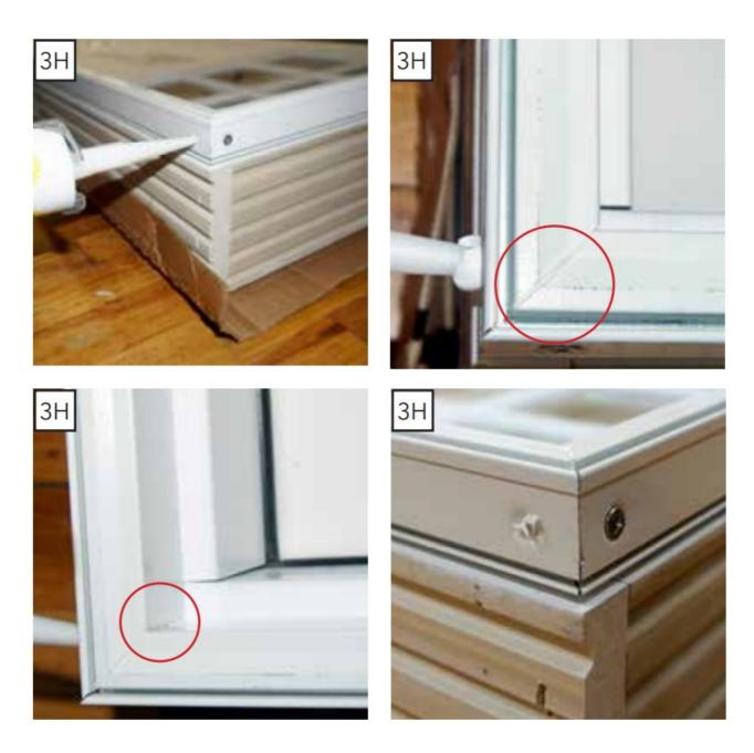
I. If there is a gap in any corner, tap on the frame near the sill to close the gap.
