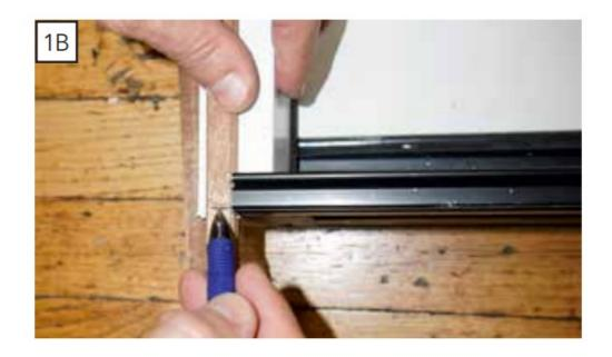
C. Cut the jamb molded nose to length.
