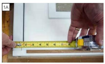
B. Keeping the molded nose in place, mark the nose at the other end of the frame 1/8" short of the sill end.
