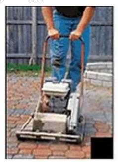
Use the plate compactor to set the pavers in place.
