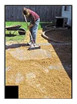
Dump sand liberally over the installed pavers and sweep it into the joints until all the cracks are filled.
