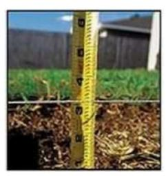
Measure the depth of your excavation frequently. Measure from the line, not from the surface of the ground.
