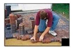
Lay the pavers working out from one corner. Keep your lines straight, and work from on top of the pavers you have already installed.
