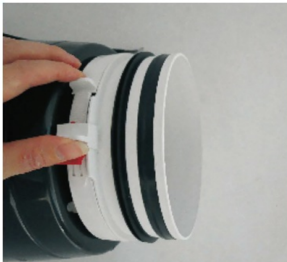
Lock the fan in place with the plastic clips
